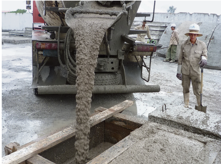
Cementing sustainability Concrete slabs made from LC3 COURTESY: PROF FERNANDO MARTIRENA, DIRECTOR, CENTER FOR RESEARCH & DEVELOPMENT OF STRUCTURES AND MATERIALS (CIDEM)
